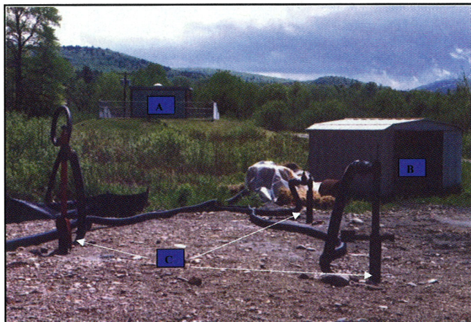
Figure 2. Locations of the existing production wells at the Tolan Farm well site. A = 26-inch by 34-inch gravel well. B = 8-inch diameter well. C = 2 1/2 - inch diameter steel cased observation wells.
