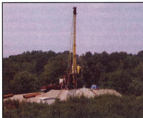
Figure 11. View of drill rig on new working surface for Tolan Farm well.
