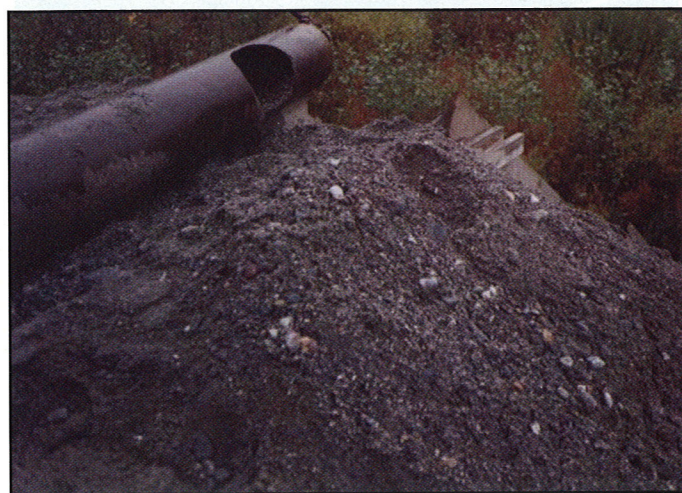
Figure 7. Gray, fine to coarse sand and gravel aquifer material removed from the well screen area during the installation of the Tolan Farm well.
